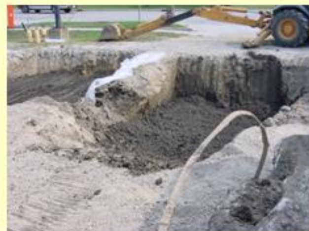
Breakage and mixing of the excavated clay
